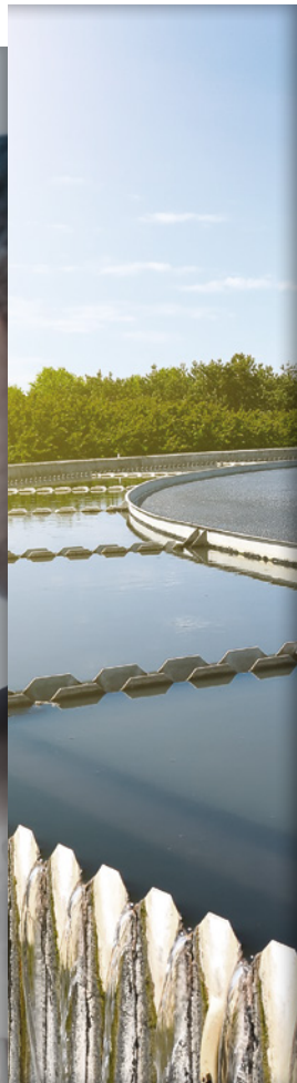
WATER AND EFFLUENT TREATMENT
